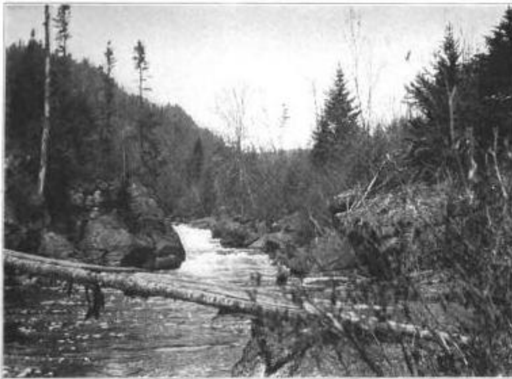
Bridge over Ste. Anne River.
